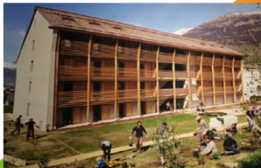
这栋大楼使用了共 15 吨羊毛，全部来自于大约 1.2 万头当地饲养的绵羊，是建筑物保温的绝佳天然材料。瑞士布里格镇圣·乌苏拉 (Sainte-Ursule) 社区公寓楼 Fifteen tons of wool from around 12,000 sheep in the region provide a good natural insulation material for the apartment building, St. Ursula community residence, Brig (CH)
