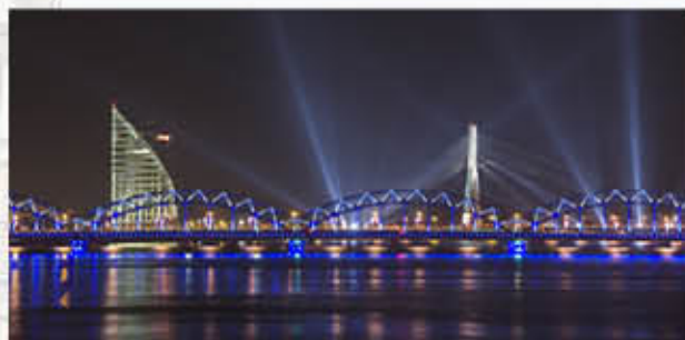
里加铁路桥 The Rail Bridge in Riga
