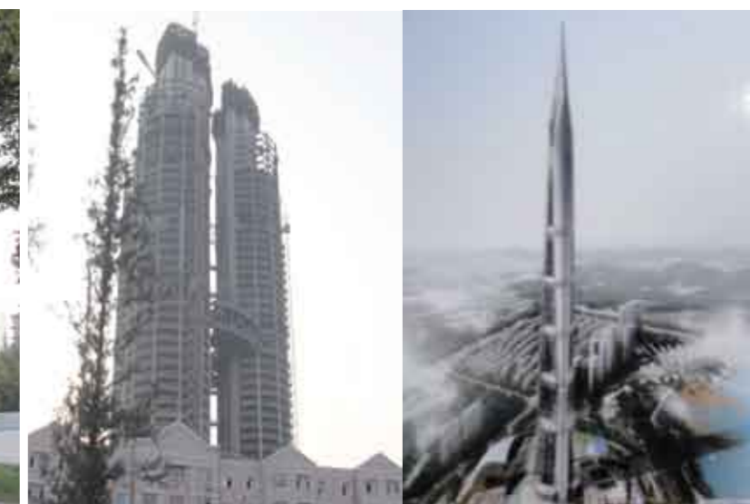
The 3 building which under construction, 328 meters high. After completion, it would be the world's first 15 high building. The total investment approach RMB 2.5 billion.
